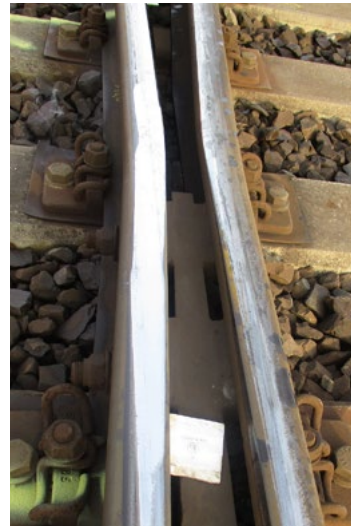
One side of a wing rail
