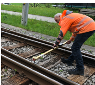
Taking measurements on a switch
