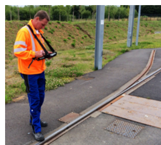
Visual inspection of switch
